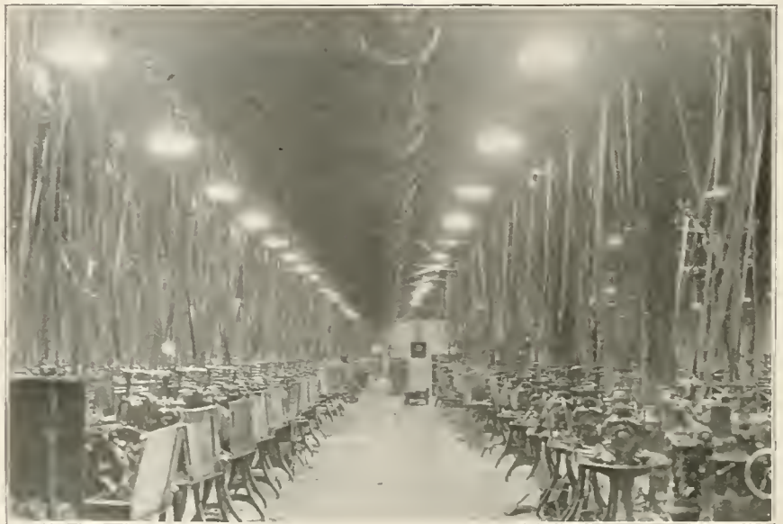
Same shop with general lighting installation made.
